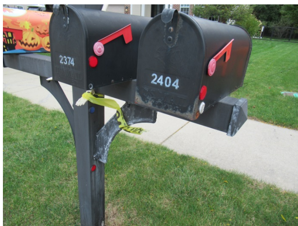
Finish deterioration
