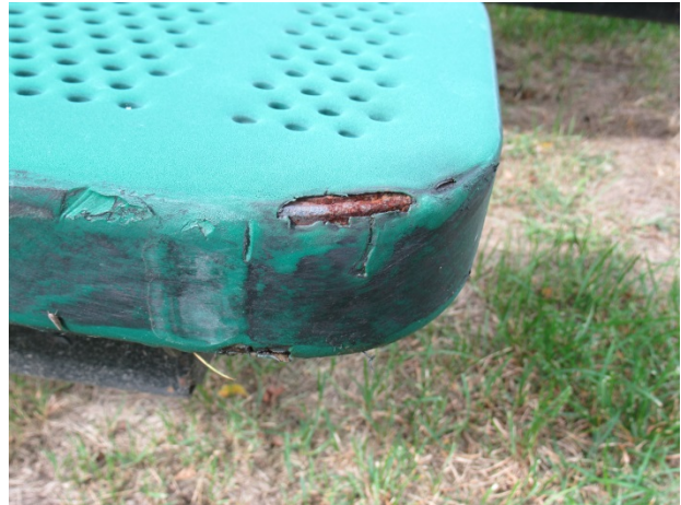
Picnic table finish deterioration and rust
