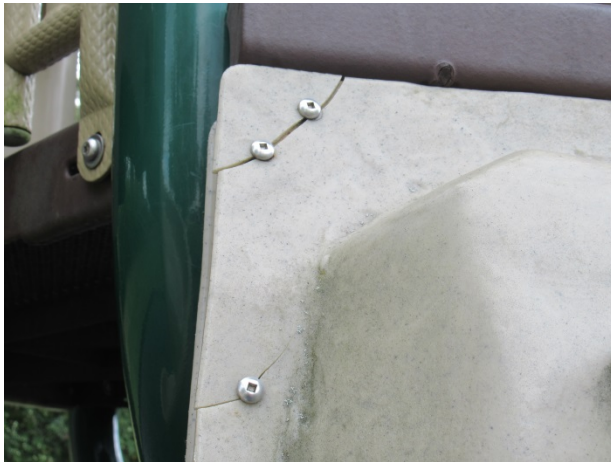
Crack at the rock climber
