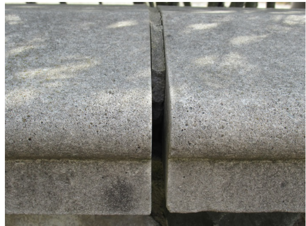
Mortar deterioration
