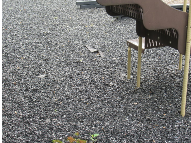
Diminished rubber mulch (note visible underlying fabric)
